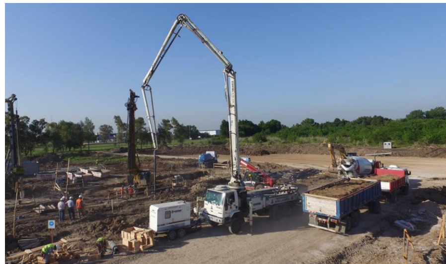
11/04/16 – Pile Driving for Turbine Base
